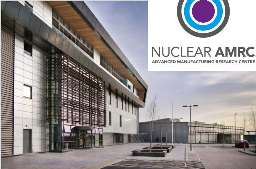
NAMRC facilities, Advanced Manufacturing Park, Sheffield, UK
